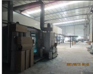
Photo of the inside of the main production hall Painting.JPG
