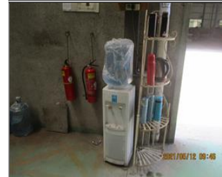
Photo of the sanitary facilities Drinking water.JPG
